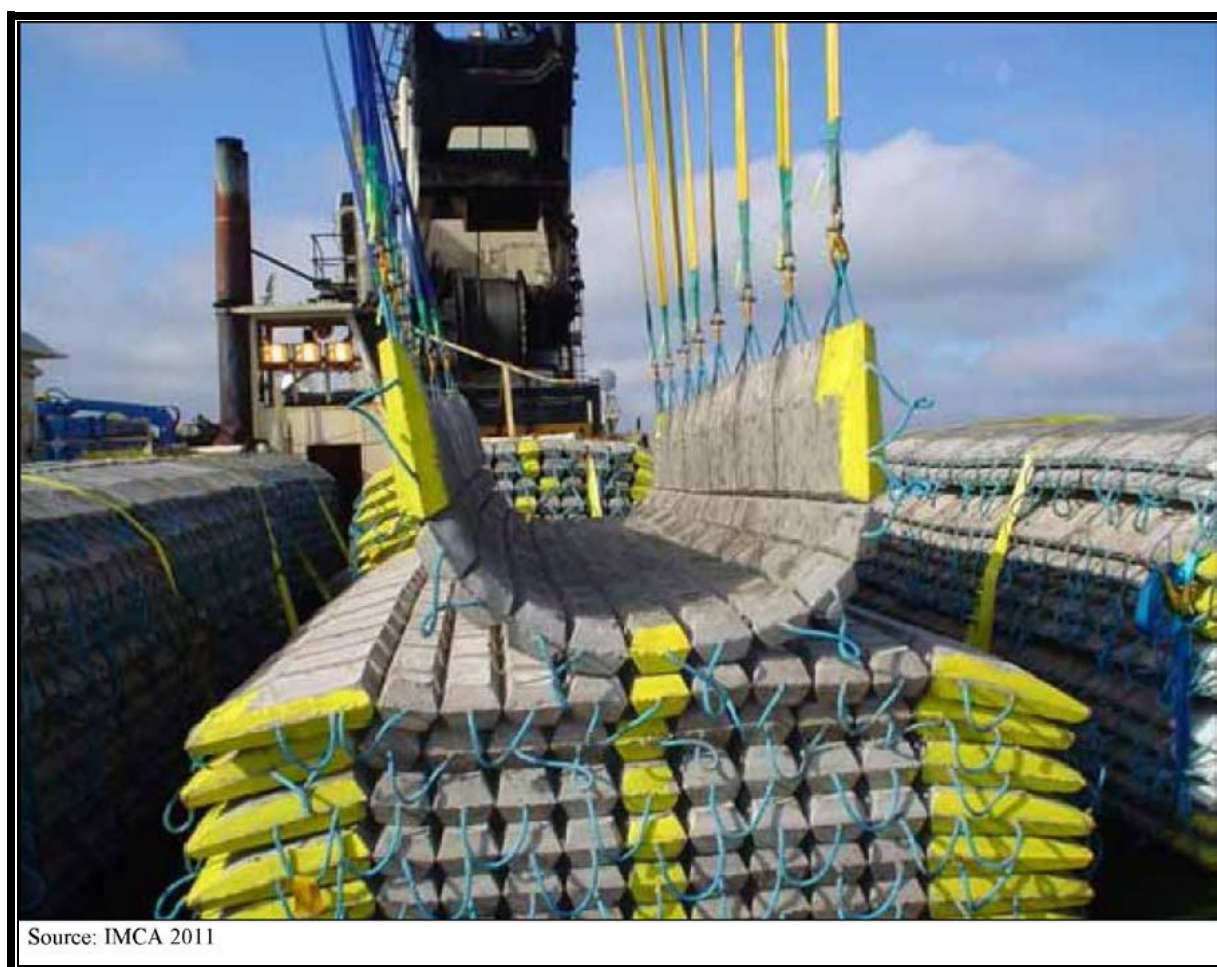
FIGURE 2-4 TYPICAL ARTICULATED CONCRETE MATS
