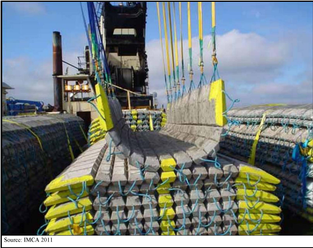
FIGURE 3-5 TYPICAL ARTICULATED CONCRETE MATS
