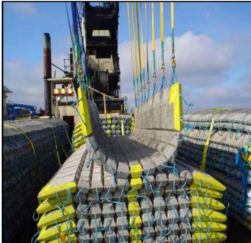
Example of a Concrete Mattress
