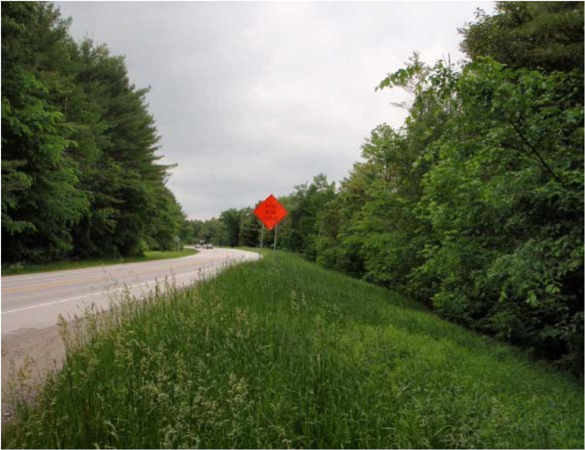
Photo 11. Typical NECPL cable route on Route 103 in Claredon, VT
