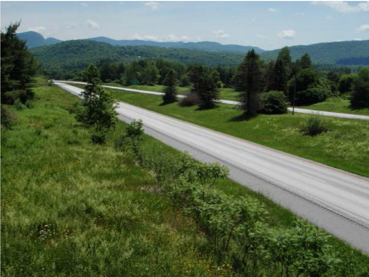
Photo 9. Typical NECPL cable route on Route 4 in Castleton, VT
