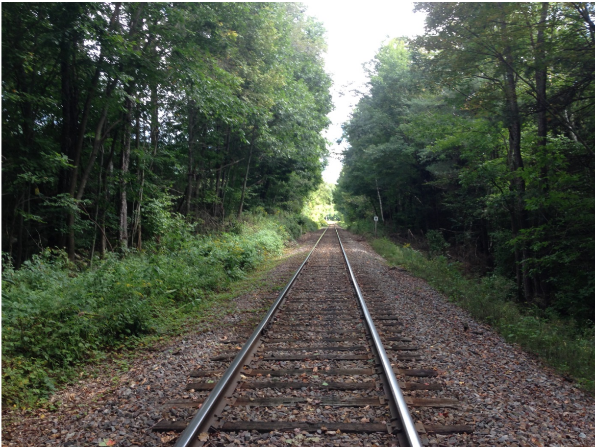
Photo 12. Typical NECPL cable route on railroad route in Shrewsbury, VT
