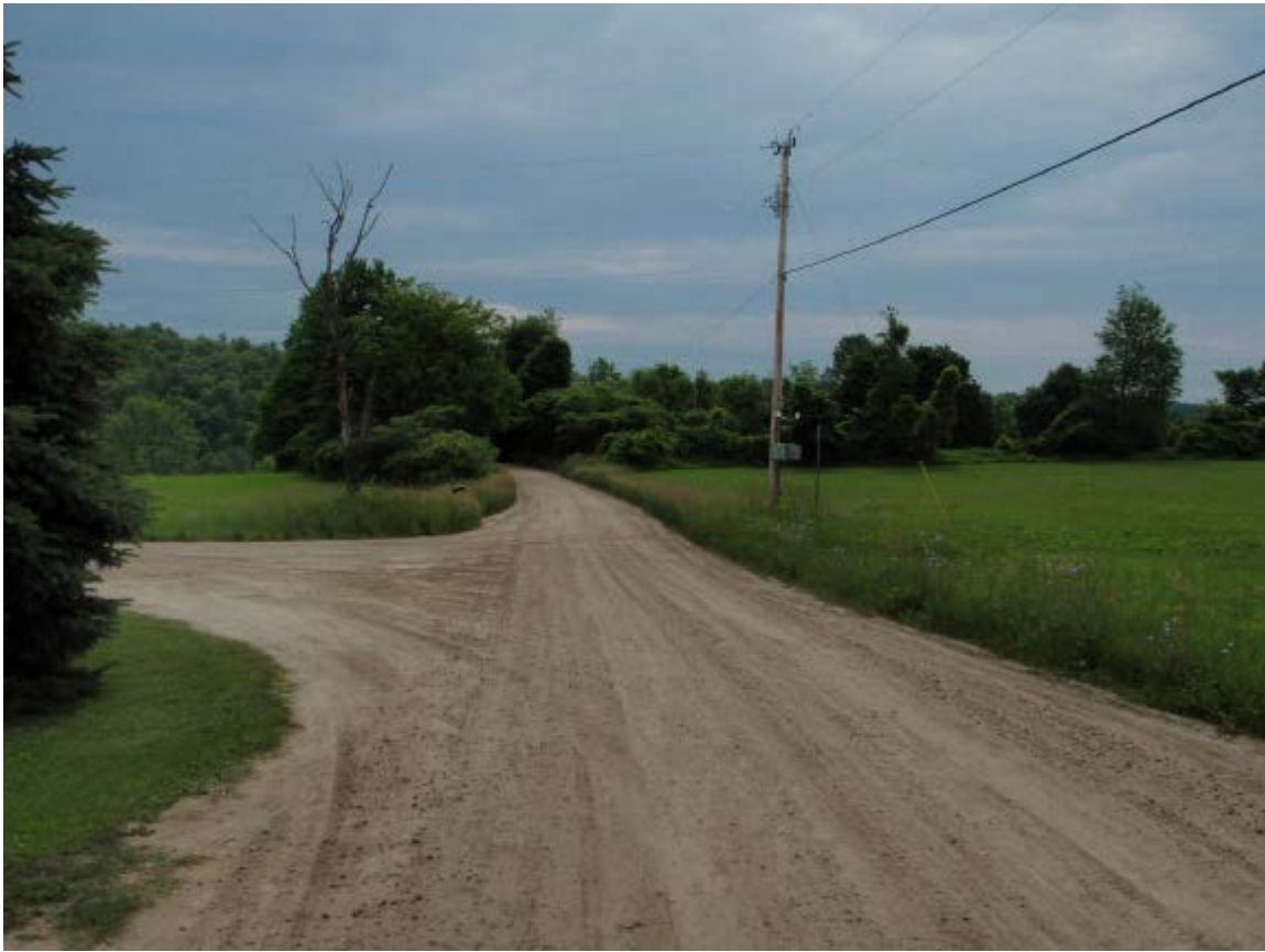
Photo 5. Typical NECPL cable route on town road in Benson, VT
