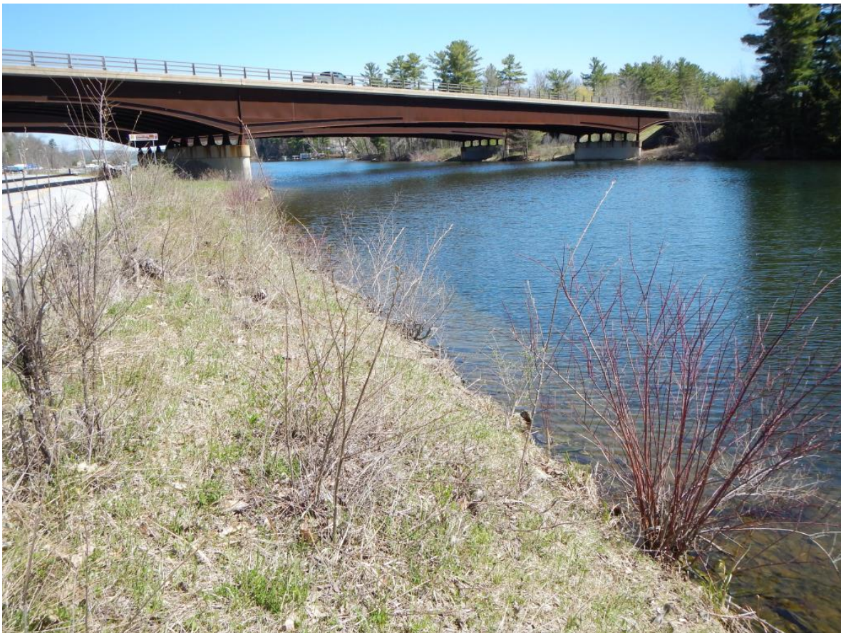
Photo 8. Lake Bomoseen in Fair Haven, VT (NECPL cable route via HDD under the lake)
