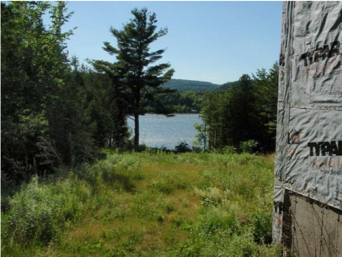
Photo 4. NECPL exit out of Lake (using HDD), from TDI-NE property in Benson, VT
